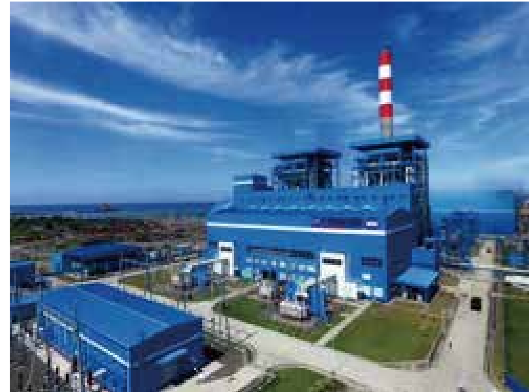
Jeneponto 2x135MW Power Plant
